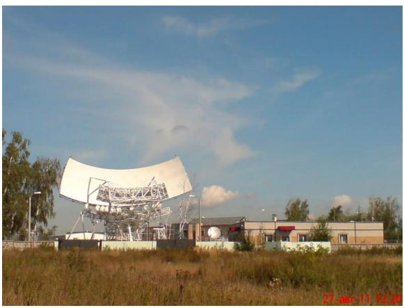
Figure 28. Russian multi-beam antenna, Klimovsk
